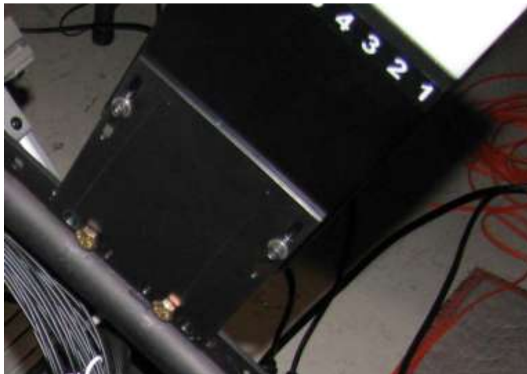
Figure 28 - USBAD mic-array mounting on gusset.
