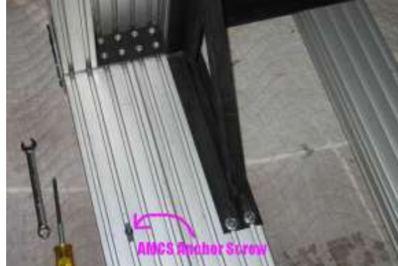
Figure 17 - AMCS Anchor Screw
