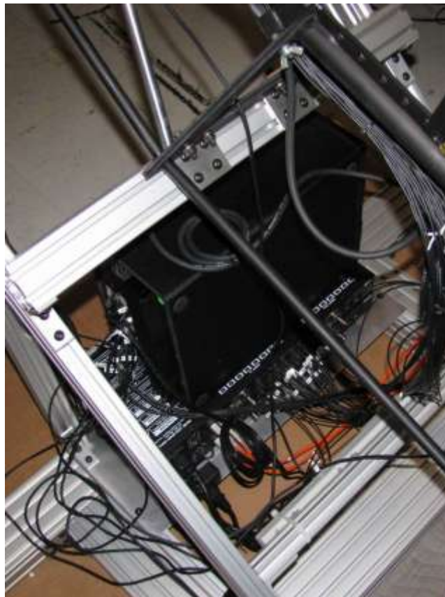
Figure 29 - Amplifier Location within truss-base.
